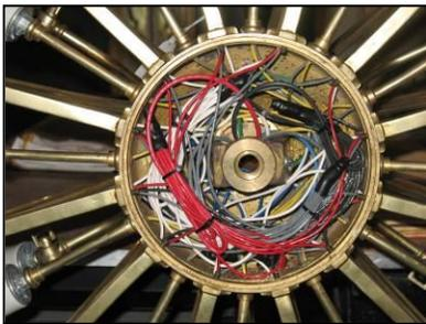
ELECTRICAL REPLACEMENT/RESTORATION/UL UPGRADING was incredibly time-consuming. Ground wires missing or not acceptably connected to the chandelier bodies, exposed wires, cloth wires held in place with wire twists, and corroded sockets all needed attention. All existing wiring was completely stripped from the chandeliers and replaced with new 105-degree C Teflon insulated wiring.
